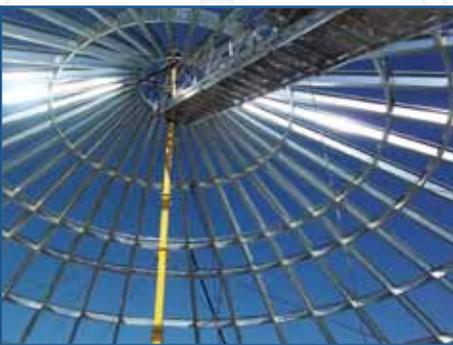
The support ring provides added strength to the roof structure. Bin/silo roofs are also equipped with 36 roof rib supports.
