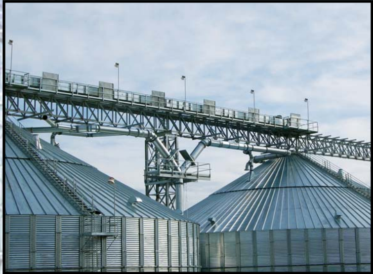
245' (74.68 m) long catwalks with 130' (39.62 m) clear span and 6' wide (1.83 m) wide Under-Truss with 10' (3.05 m) wide deck support designed for high capacity grain handling.
