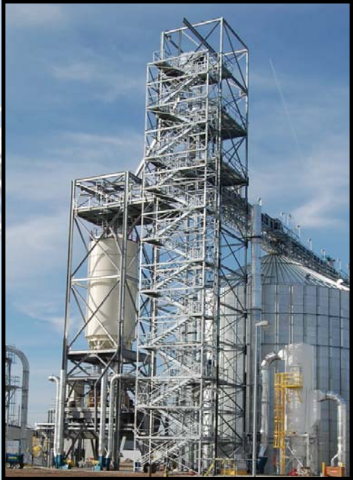
20' x 20' x 136' (6.10 m x 6.10 m x 41.45 m) Structural tower with self supporting switch-back stairway.
