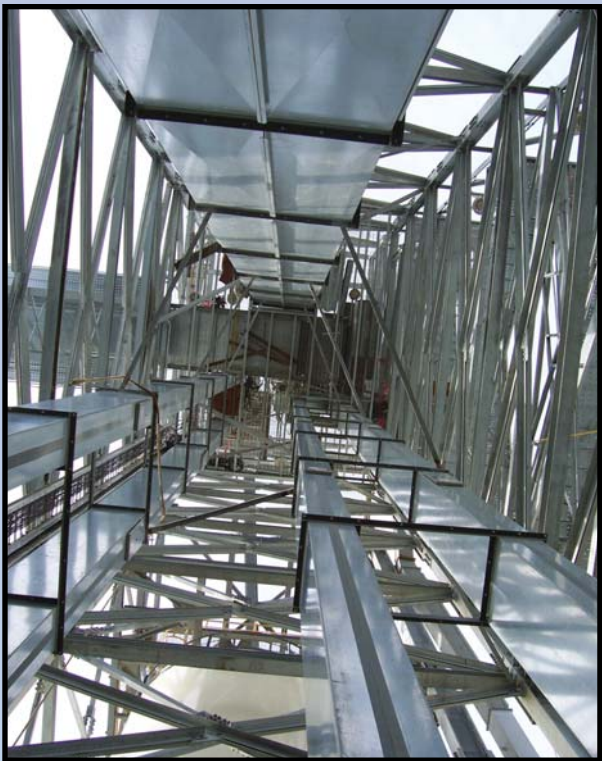
Equipment Support tower constructed with structural steel columns, beams and braces.
