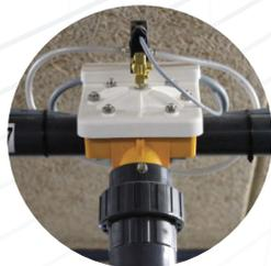
The new DM5 feed valve of datamix has been developed to withstand future demands of secure operation and easy service. The valve is equipped with a stainless rough-boring angle and stainless bolts, which makes it easy to dismantle. The rubber-diaphragm is made out of 2 layers of rubber, which are vulcanized around a heavy fibre-net. This assures a powerful diaphragm with optimal life span.
